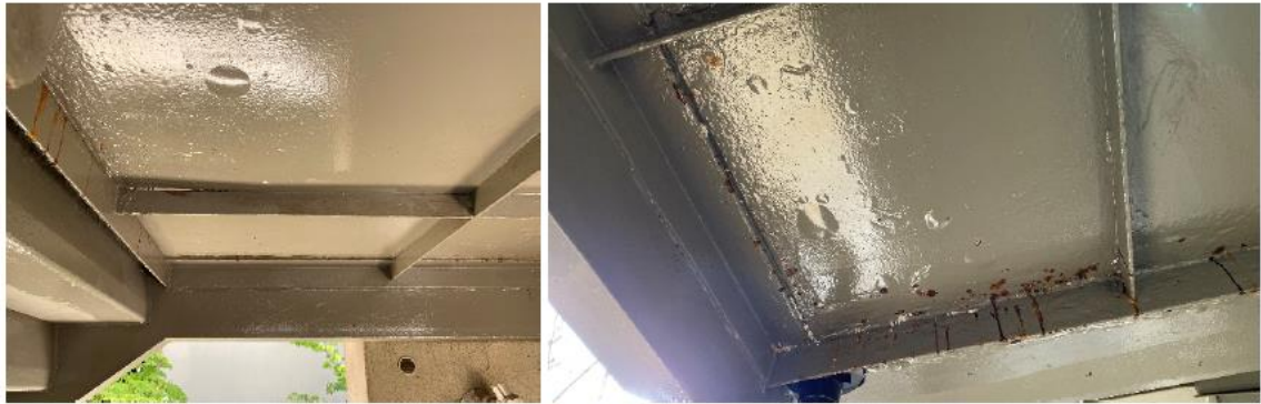
Figure 7 - Rust bubbles and corrosion streaks
