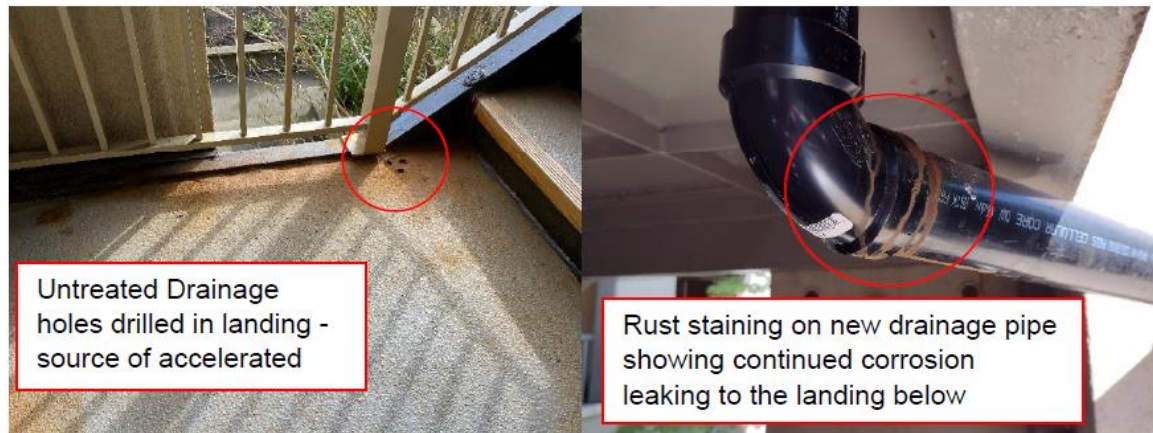
Figure 3 - Accelerate rust caused by new, untreated drain holes
