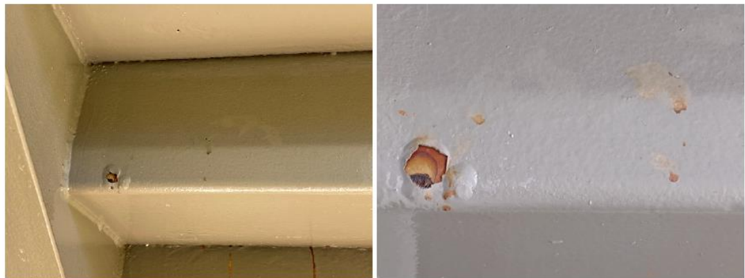
Figure 6 - Rust bubbles broken through, evidence of repair/repainting since restoration
