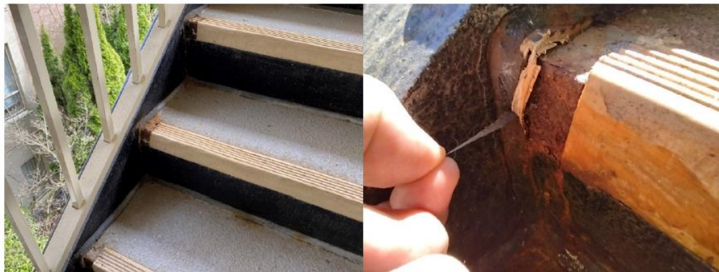
Figure 2 - Stair deck surface left unrepaired and exposed. Accelerated corrosion in need of immediate repair
