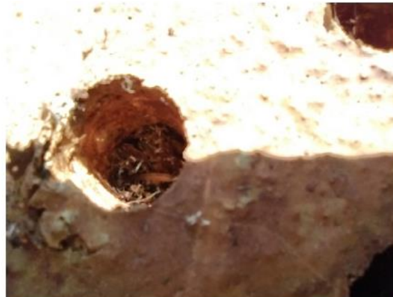
Figure 4 - Unprotected drain holes clogged with debris continue to flood landings
