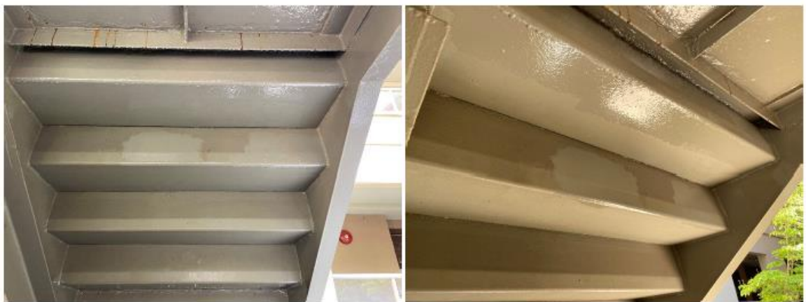
Figure 1 - Mismatched paint showing repairs have already been completed since restorative maintenance concluded
