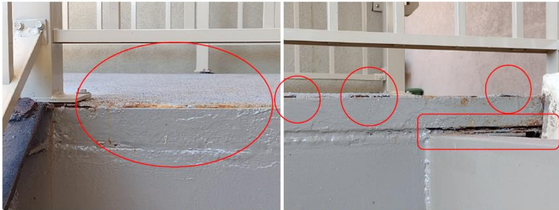
Figure 5 - Raised deck surface membrane lifting, rusting, lack of sealing - East Staircase
