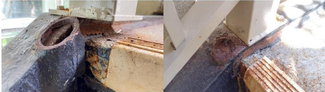
Figure 1 – Incomplete repair allowing accelerated corrosion in need of repair (Central stairs – left, East Stairs – right)
