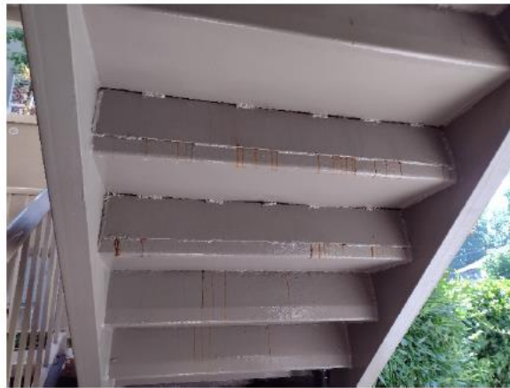
Figure 8 - Rust streaks from subsurface corrosion continue to this day
